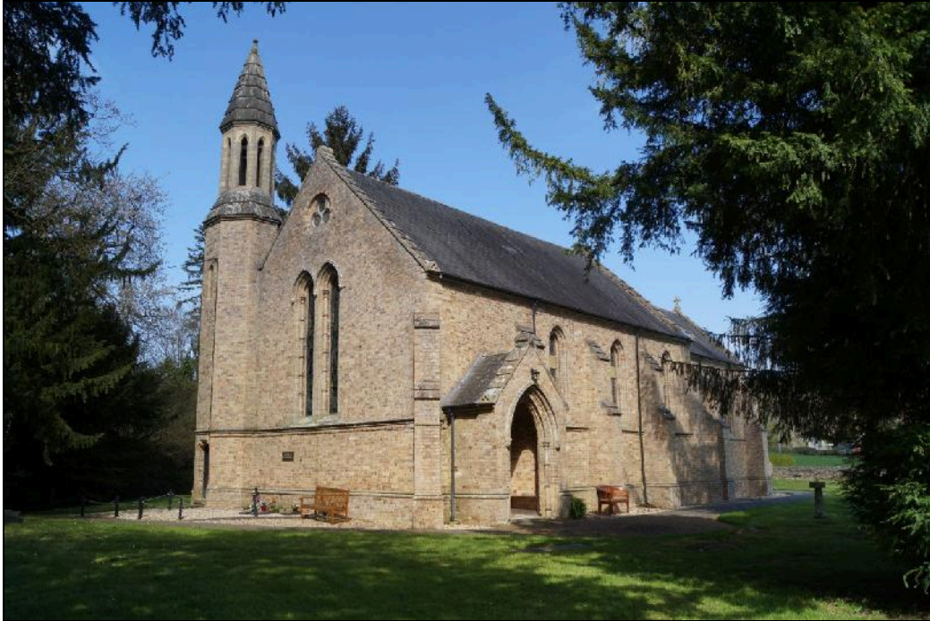
Plate 27: Probably the best view of the church from within the churchyard (SJ23653 16574), April 2019, shows that the church and churchyard trees block any view towards Penrhos Farm and the new steel frame building. This is a key view of the church from where it can be appreciated and understood. Looking northeast.
