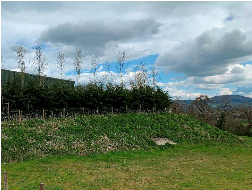
Plate 38: A view of the bund around the southern end of the new steel frame building at Penrhos Farm, April 2021, showing the screening trees growing along the top of the bank with additional deciduous trees planted alongside the Leylandii hedge. Further trees will be planted in front of the bund in future. Looking east-northeast.
