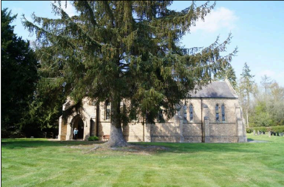
Plate 23: A view towards Penrhos church from the same position as Plate 38 (SJ23679 16567), April 2019. This is a good view of the church, but not one in which it can be well understood and appreciated as the large conifer in the foreground blocks much of the view. The steel frame building at Penrhos Farm does not have a significant impact on this view but is in the periphery of the viewers' eyeline not shown by the camera. Looking north.
