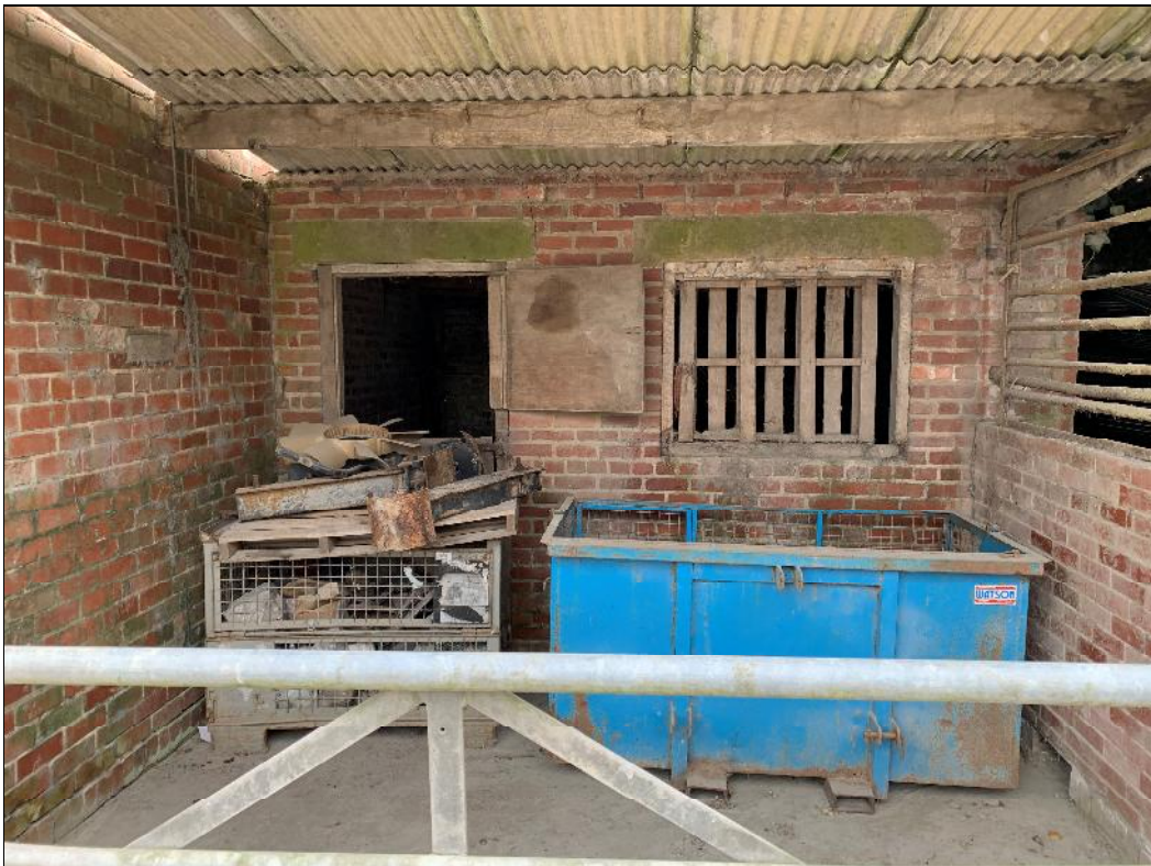
Plate 12: A view of the possible dog kennel in Building ID number 41 in Deytheur Yard. Looking south-southeast.
