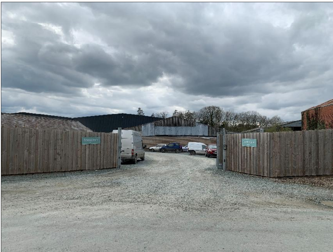
Plate 8: A view of the entrance into Penrhos Farm with the eastern gable of Building ID number 40 at the centre. Looking west-southwest.
