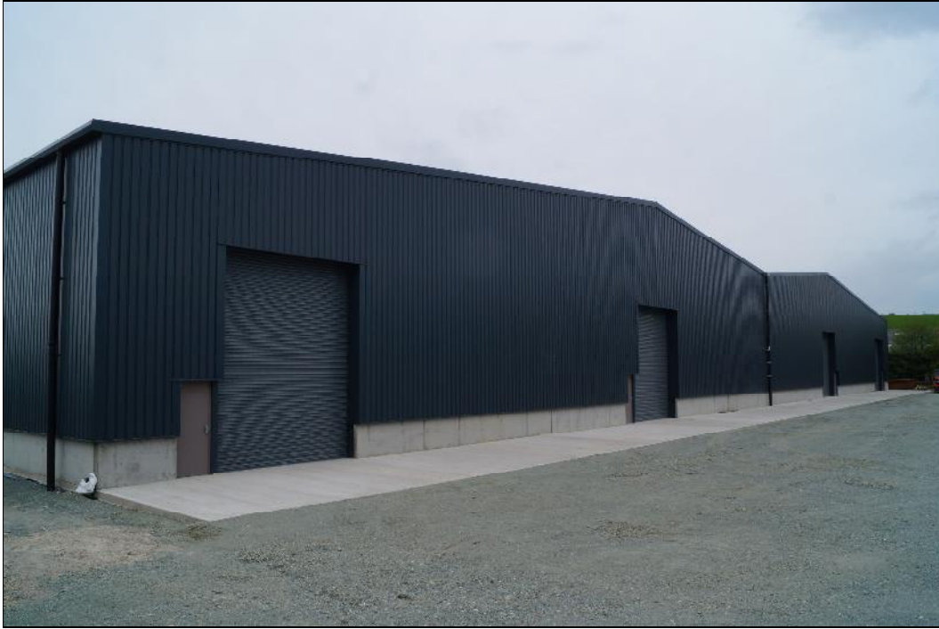
Plate 1: A view of the new storage shed at Penrhos Farm, painted dark blue-grey, May 2018. Looking northwest.
