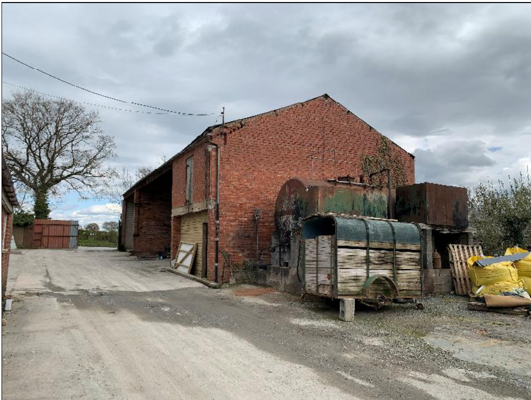
Plate 10: A view of Building ID number 38 in Deytheur Yard. Looking east.
