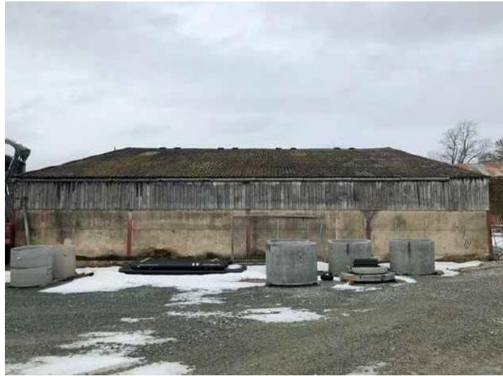
Figure 2-1 Image of the previous structure
