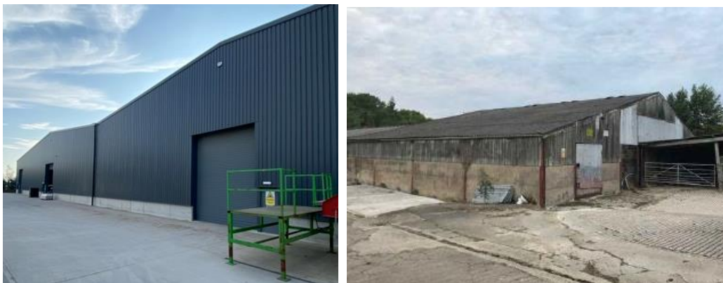
Figure 3-1 Picture of old and new warehouse
