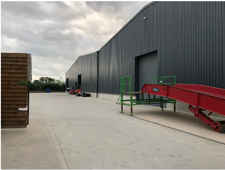
Photo 1 Steel portal frame building in use for storage, showing east elevation with entrance bays and hardstanding for servicing
