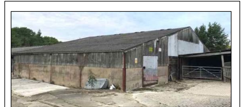
Photo 1. View of east and south façades of existing barn
