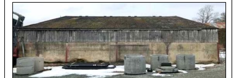
Photo 2. View of south façade of existing barn
